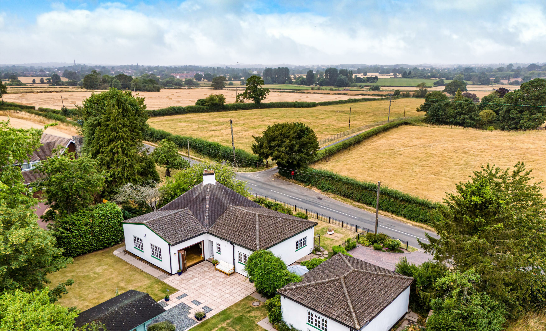
1 Claygates Bungalow, Crateford Lane, Nr. Brewood, Stafford, ST19 5PZ
